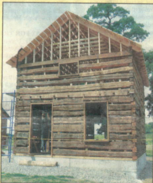
CABIN FEVER — On Wednesday, volunteers added the board and battens on gable ends to the restored 1850s two-story log home being reassembled in Dorothy Carnes County Park outside of Fort Atkinson. Seen here are pictures from the construction site. Above, volunteer Greg Idzikowski takes a breather during the work day. At left, the structure gets closer to completion. At right, Jefferson County parks operations supervisor Kevin Wisemann notes the wire meshing that will be used to hold up a mortar mixture between the logs. Related photos appear on page A3. — Daily Union photos by Paris Knox.
